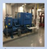
Tecogen air conditioning chillers operate without significant electricity requirement sidestepping utility demand tariffs
