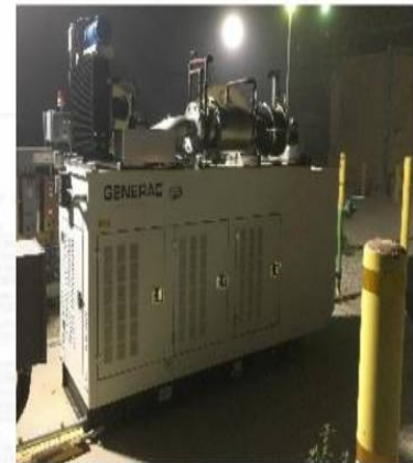
Natural Gas Generator Upfitted with Ultra in Southern California (LA County)
