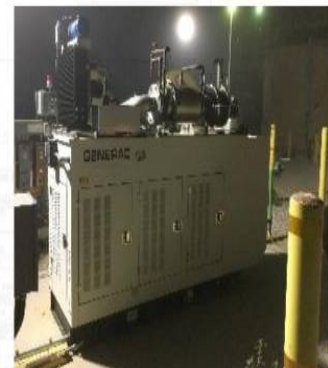
Natural Gas Generator Upfitted with Ultera in Southern California (LA County)
