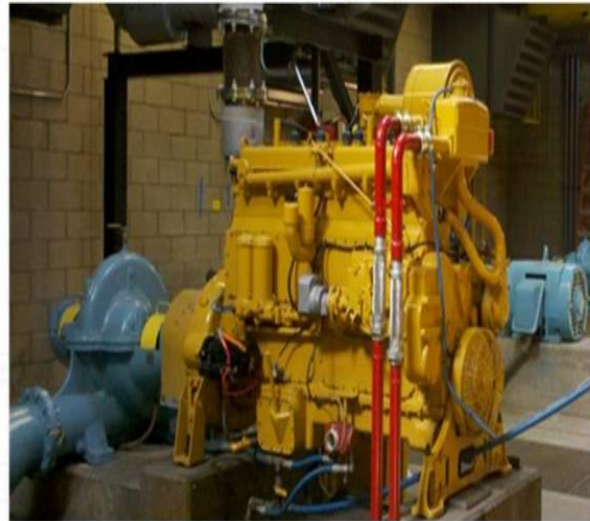
Ultra equipped 300 HP water pumping natural gas engine
