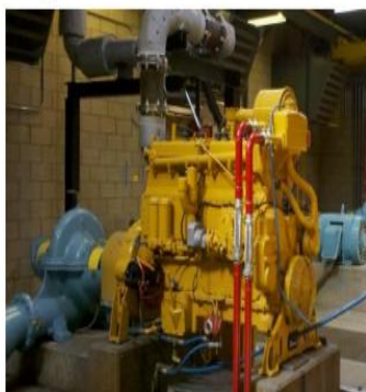
Municipal Water Pumping NG Engine – 250 HP
