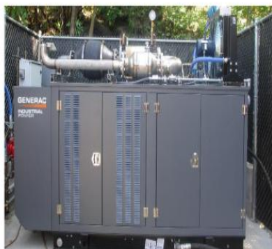
NG Emergency Generator 100-250 kW
